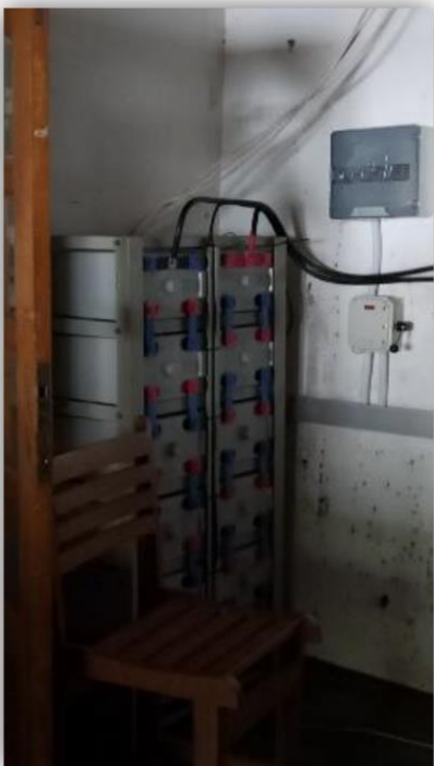
Solar panel transformer 2017 – Interior view
