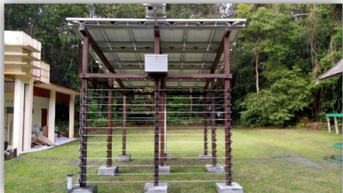
Solar panel installation 2017 – Exterior View
