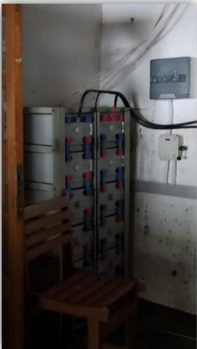
Solar panel transformer 2017 – Interior view
